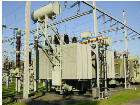
HS/MS-transformator
