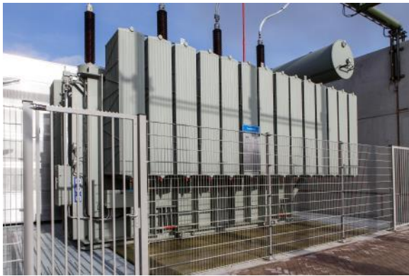
HS/MS-transformator
